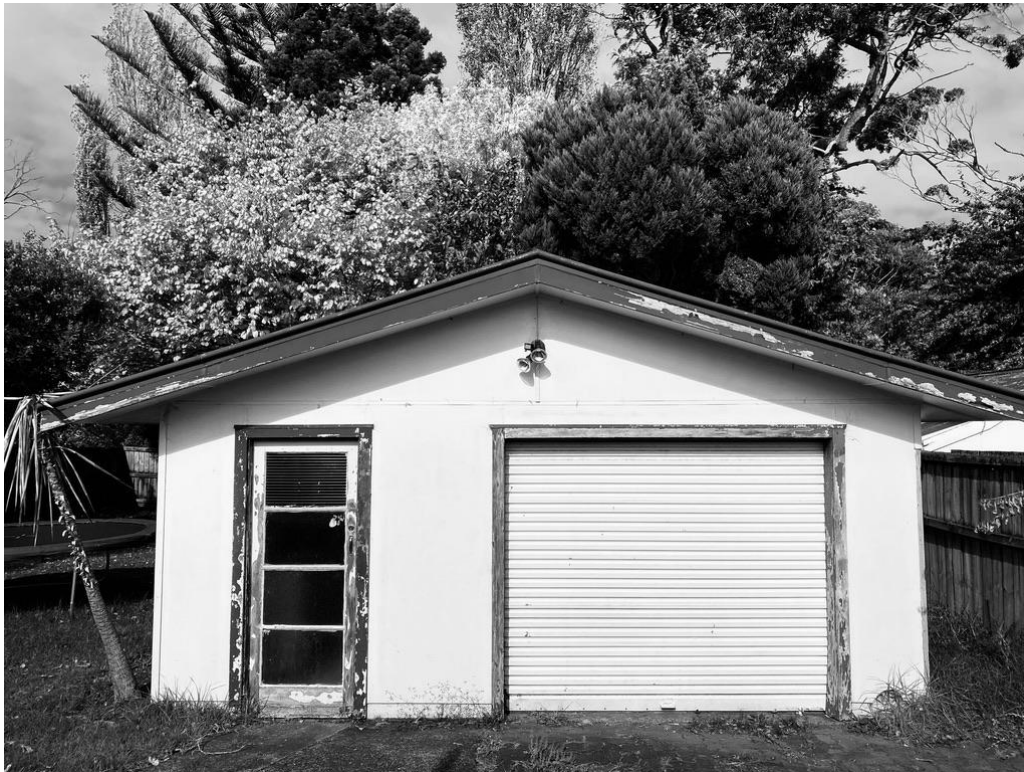
The site of Vunilagi Vou 2.0, before refurbishment. March 2020.
